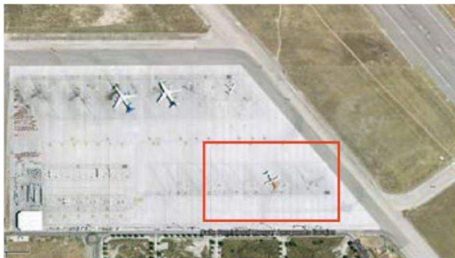
Solera intervenida con SOIL STABILIZATION GEOSEC
